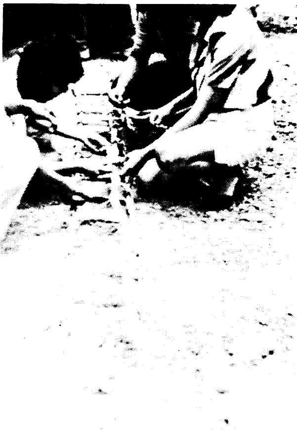
Figure 37. Students from the Architectural School of Laica University building a frame of braided bamboo cables for use in a concrete beam.
